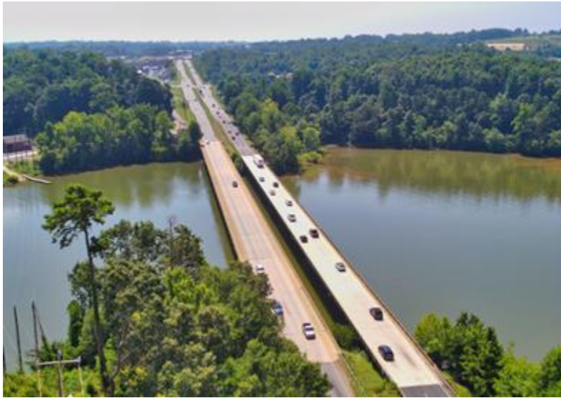
Figure 2: US 321 Bridges Over Catawba River
